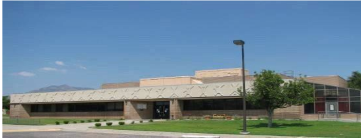
School Age Care (Bldg. 1316) (575) 678-4140
